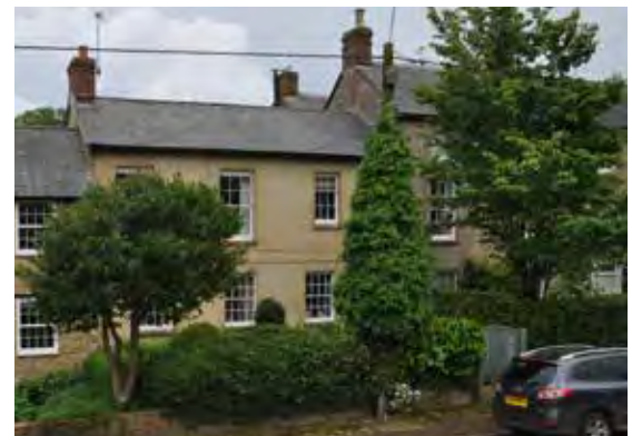
Dower Lodge may have been single storey. The elevation facing the street has stone coloured render struck as stone.
