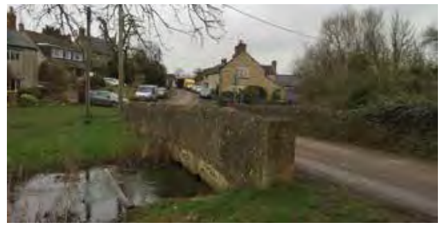
Bridge over the brook from the north looking east
