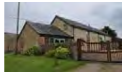
The Threshing Barn
