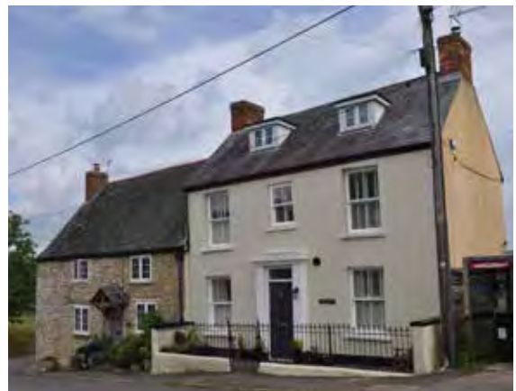
Springhill House has received a modern render which is painted to the front.
