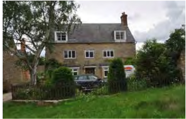
Hethe Cottage (Hospital Farm)
