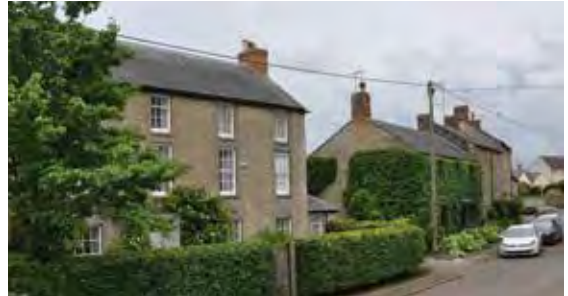
Hethe House is 3-storeys high with a roof pitch built for slate.
