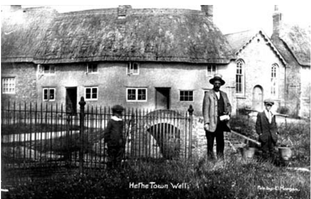
Originally 3 cottages: note the eaves height, the thatched roof and balanced flush casement window design on Knowle Cottage. The high proportion of solid wall to void opening is traditional in vernacular cottages in the district. Postcard 1900-1910. Copyright: OCC/E Morgan
