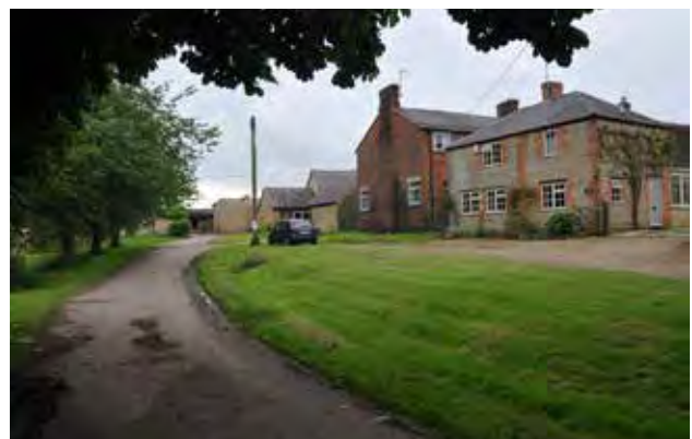
Former farm buildings to the west of The Green have been converted to housing
