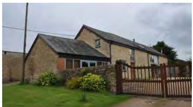
The Threshing Barn
