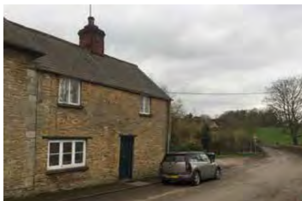
7 Main Street, with its ad-hoc window arrangement and high proportion of solid wall to openings
