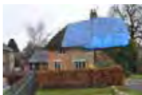
The Old Carpenter's Shop
