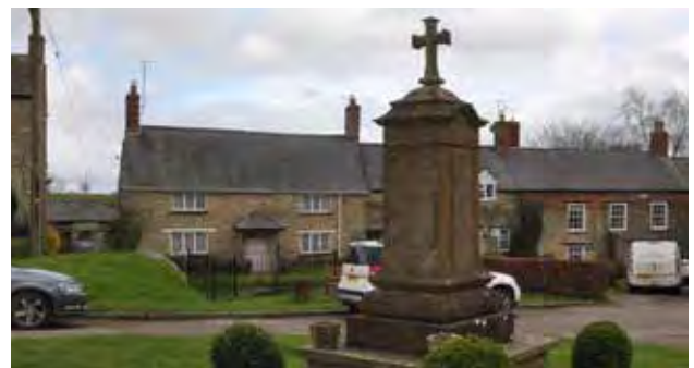
The timber windows and doors have been lost and a different porch has been added.
