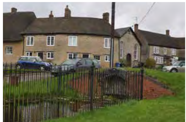
The three cottages are now in single ownership: Bow Cottage. The painted timber doors and window casements have been lost and the first floor windows have increased in size, as the eaves have been raised. The elevation now looks top heavy. The thatched roof has been replaced by tile. The gable chimney on the Old Post Office has been lowered.
