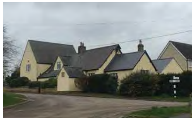
The school has been converted to a house. The school has been much extended and the masonry is now rendered.
