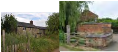
Fir Tree Cottage, outbuildings and walls
