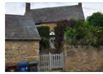
Hedham House (formerly Goldhill Cottage) and outbuildings.
