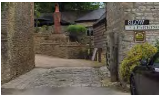
Aesthetically pleasing cobbles at the entrance to pub car park also warns drivers to slow down
