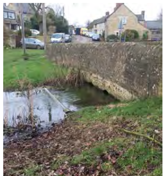
Water level of Hethe Brook under the bridge looking east, March 2020
